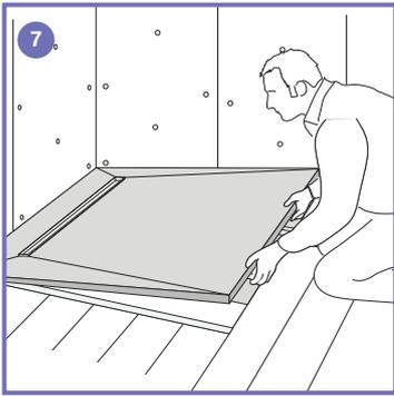
7. Position the shower base over the drain to make sure they are correctly aligned. (But don't remove the protective cover and force the nozzle in to the drain). Ensure any connections created are waterproof at this stage because it will not be possible to return to them once the unit is tiled. (You can do this by pouring water down the drain to check the seals).
